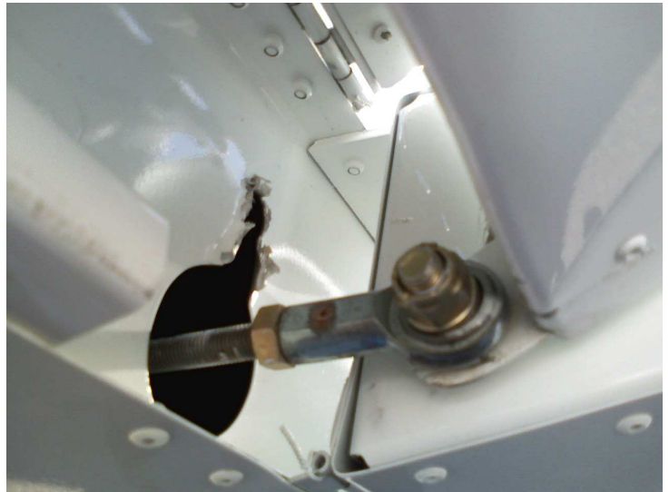
Above – Rear spar damage
